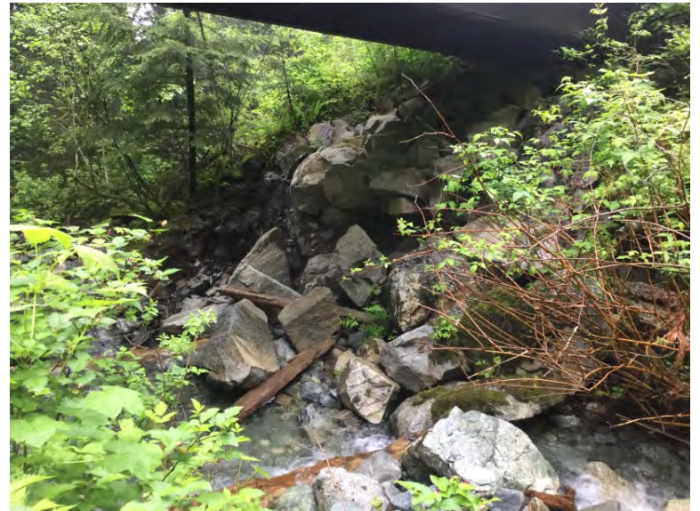
Right Bank Abutment when facing downstream
