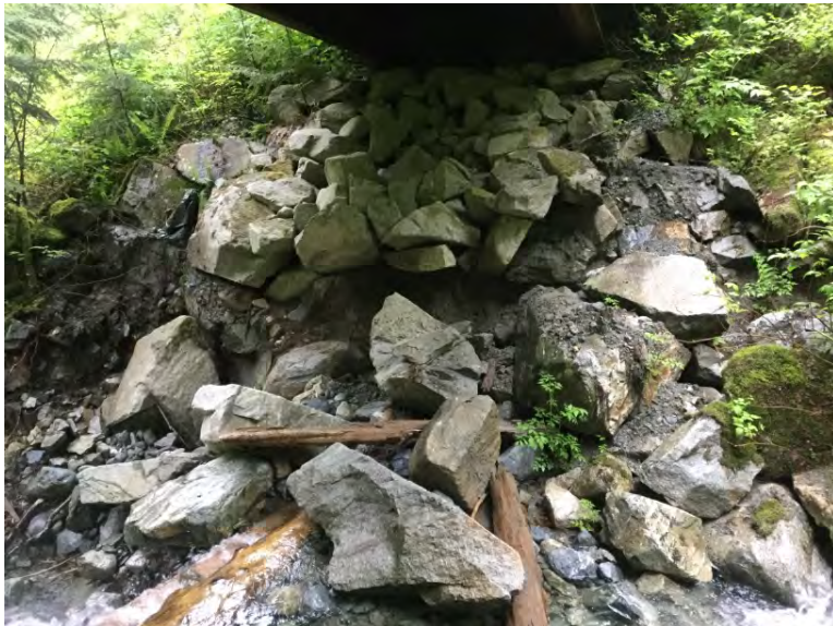
Right Bank Abutment when facing downstream
