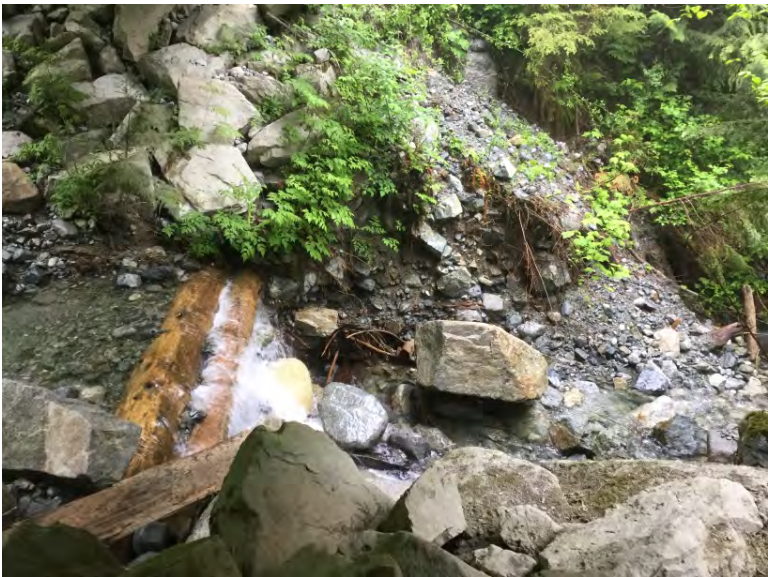
Downstream left bank scour
