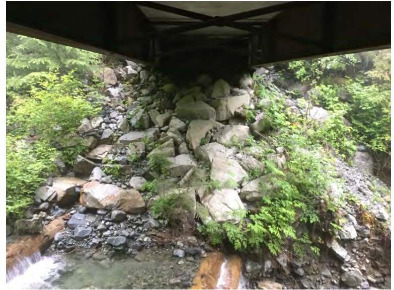
Left Bank Abutment when facing downstream
