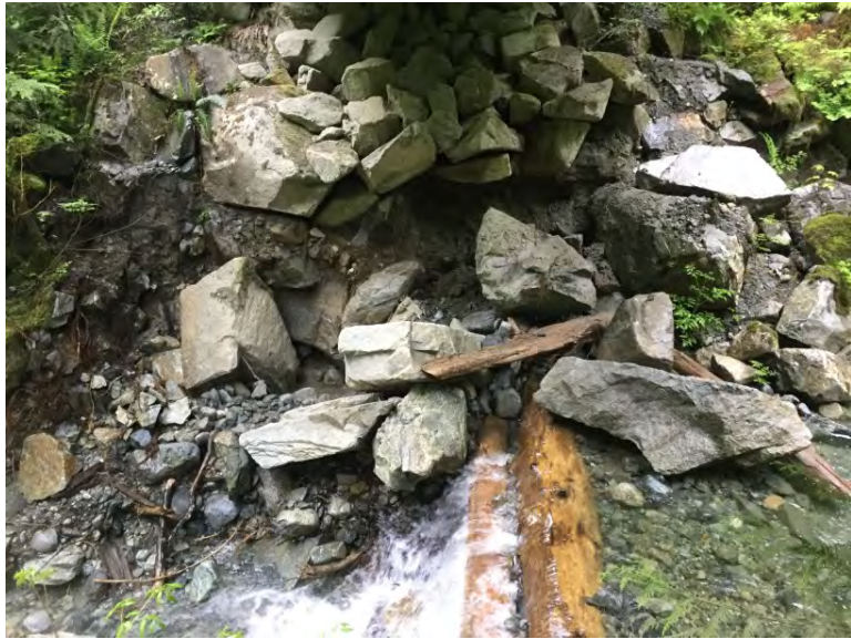
Right Bank Abutment when facing downstream
