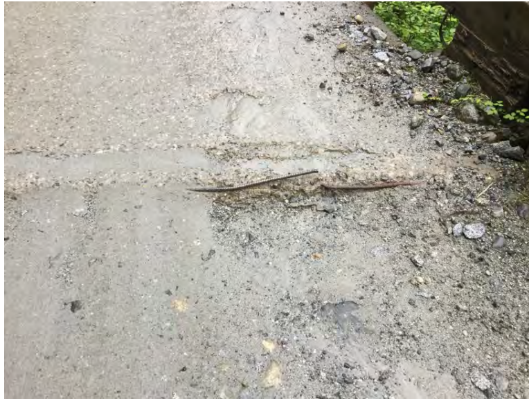
Downstream right bank ballast wall condition
